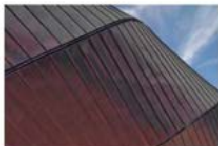
Double lock standing seam in copper
