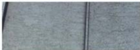
These dark spots will gradually disappear as the weathering proceeds.
