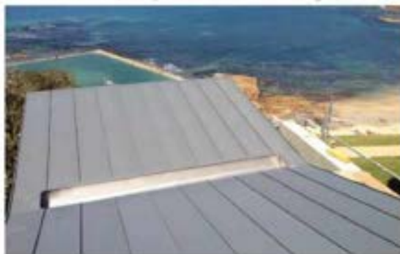
Frequently rain-washed areas do not allow salt deposits to build – eZinc Gate at Fairlight, Sydney
