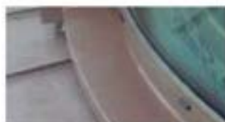
Aluminium window frame sealed against the elZinc Rainbow Brown sill using brown neutral curing silicone
