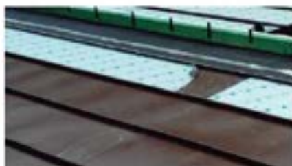
Partial removal of protective film causing marking of Rainbow brown – this can be wiped away.
