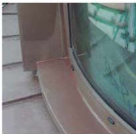
Aluminium window frame sealed against the elZinc Rainbow® Brown sill using brown neutral curing silicone
