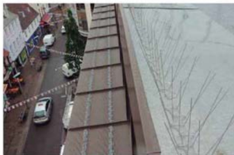
Bird spikes attached using neutral curing silicone
