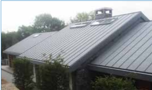
350m 2 of VM Zinc plus on Metdeck158 on plywood deck
