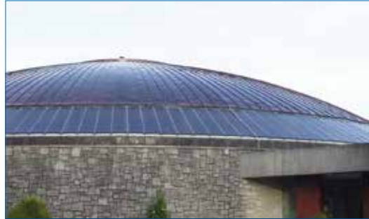
550m 2 of Classic Copper on Metdeck118 on CLT
