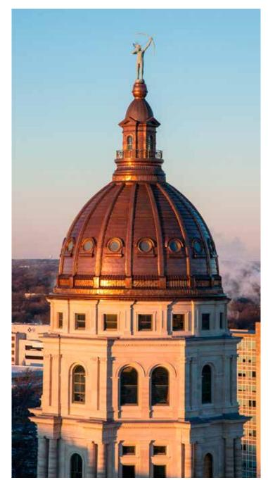
In addition to these panels, the dome incorporated new copper window surrounds, stainless steel gutter frames, heat trace, roof drains and lightning protection
